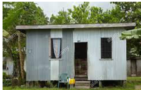
Tin /corrugated houses
