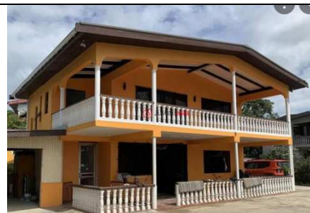
Double storey building
