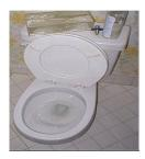
2. **Water Sealed Toilet** - is like a regular cistern flush toilet except that the water is poured in by the user, instead of coming from cistern above.
